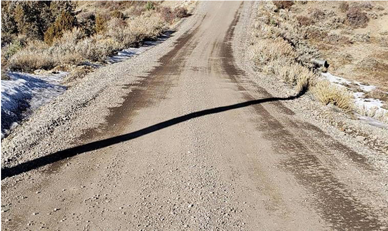
Photo of a gravel road made more susceptible to moisture damage by gravel being snow plowed into the ditches.
