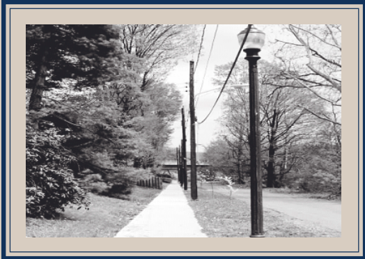
New Sidewalk and Street Lights on West Edgar Avenue in Ronceverte
