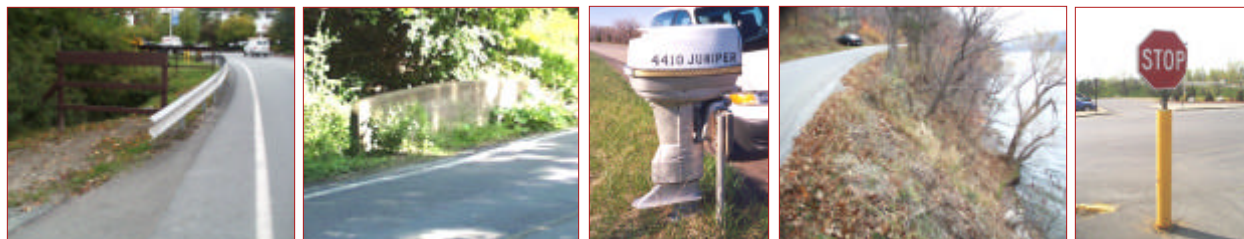
Figure 1: Common roadside hazards include unprotected guiderail ends, headwalls, mailboxes, slopes, and improper signposts
