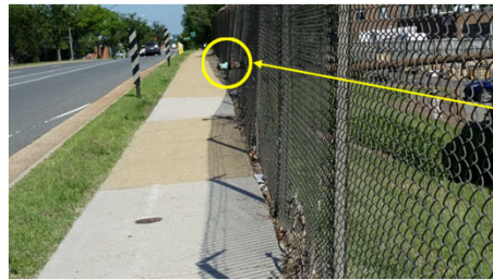
Fire Department Connection
