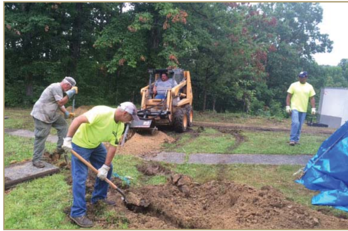
City of Philippi Public Works employees providing assistance in Bomont, WV.
