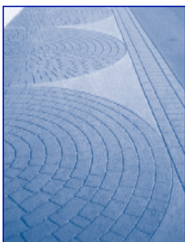
An aesthetically pleasing and realistic looking example of pavement stamping used on a neighborhood sidewalk.
